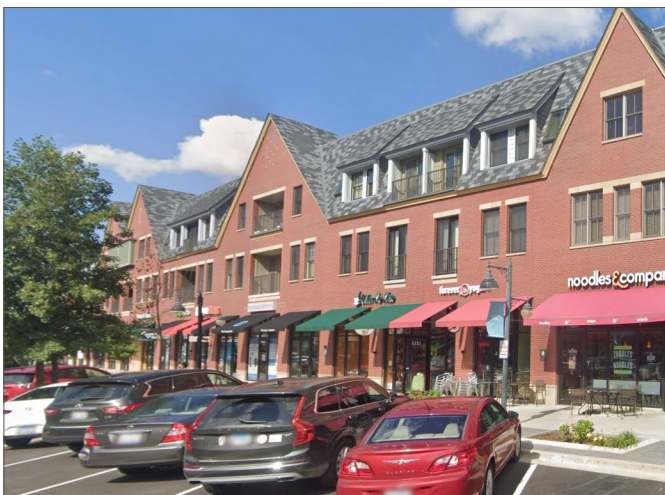
Figure 3. Examples of Village Shopfront Buildings
