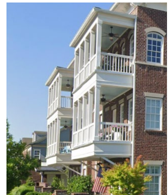
Stacked balconies with visible support structures.
