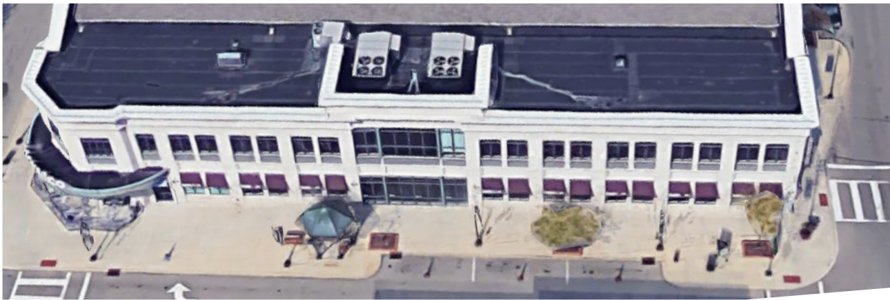
Figure 27. Rooftop Utilities Screened from the Public Way by a Parapet
